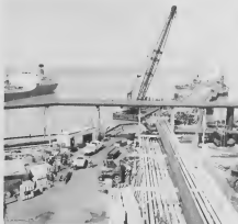
Huge crane and barge assist in recent No. 3 Finger Pier turnaround.
